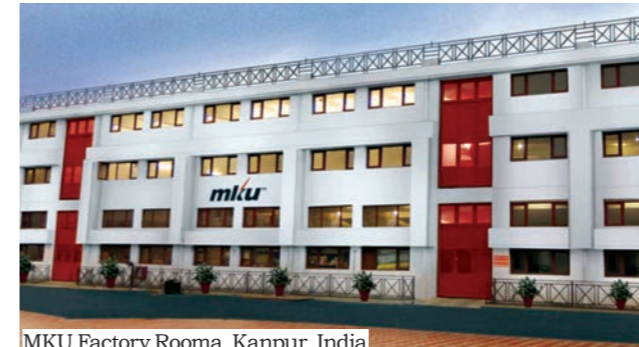
MKU Factory Rooma Kanpur India
